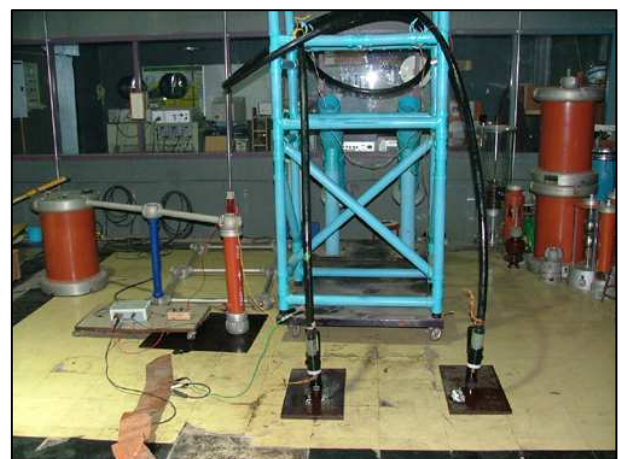
Figure 10: Show the circle of line connection which is using gas SF 6 to be insulation testing for finding the partial discharge value in the high voltage cable in the side of 24 kV
